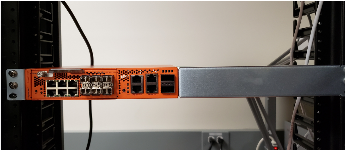
Figure 7 Four-Post Rack Installation (Single Chassis Assembly)
